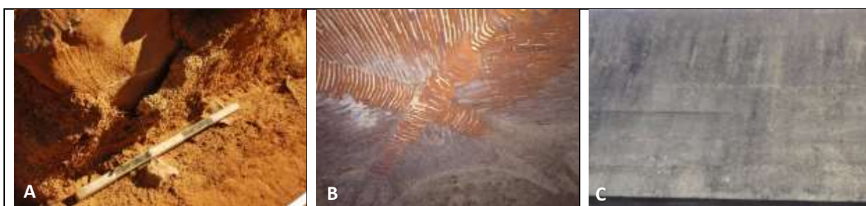
Figure 1. Envelope materials in the Portuguese built heritage: A, earthen mortar at Roça do Casal do Meio, a pre-historic site near Sesimbra; B, ceramic brick masonry ceiling in Palácio Vale Flor, Lisbon; C, concrete façade on Gulbenkian Foundation headquarters, Lisbon
